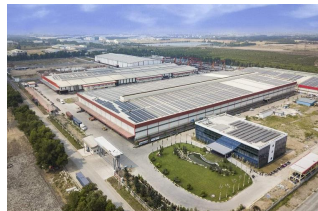
WWB(株) 海外事業 Dai Dung An Ha Factory roof top(Thang Long Power) Unnamed Road, Bình Chánh, Vietnam
