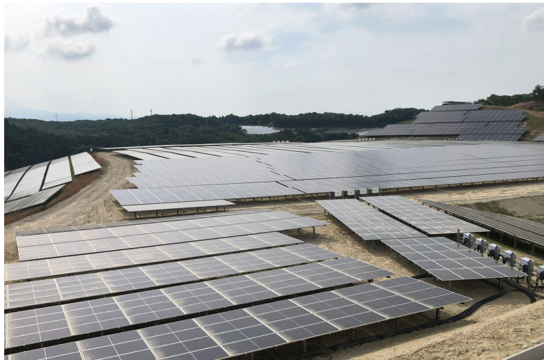
[Taiwa Town Solar Power Plant]
