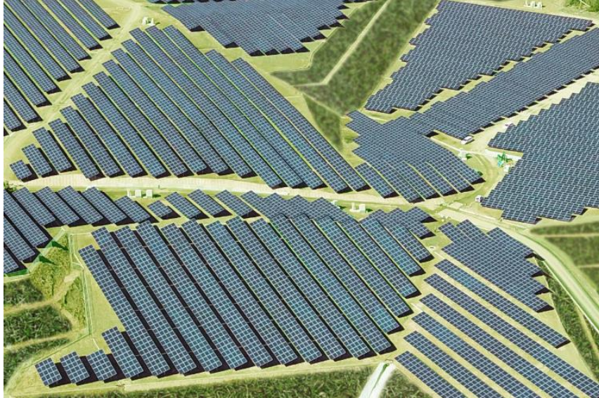
Kakuda Solar Power Plant (Miyagi Prefecture) (DC): Approx. 18.3MW
