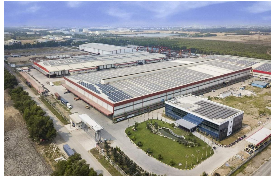
Dai Dung An Ha Factory roof top (Thang Long Power)/Vietnam
