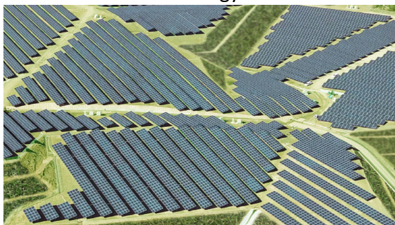
Kakuda City Solar Power Plant/ (DC) 18.3MW
